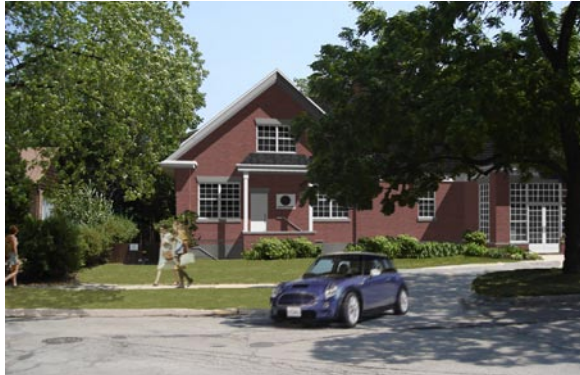
repaired + remodeled bungalow
